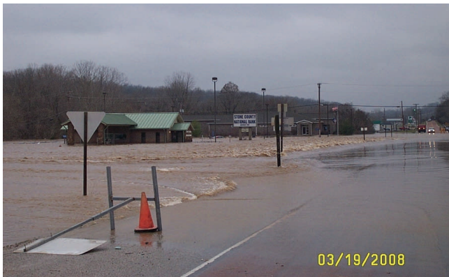
Stone County National Bank was engulfed by rising waters on Highway 413 West in Galena.
