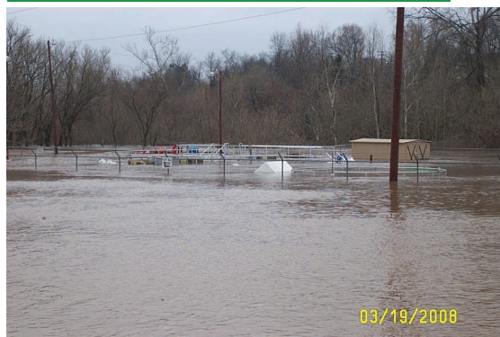
The wastewater treatment plant under water in Galena, Missouri.
