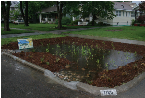
One of the Partnership's demonstration rain gardens, located in Springfield, Missouri.
